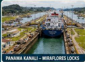
PANAMA KANALI - MIRAFLORES LOCKS
